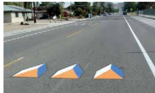
Heed the Speed safety campaigns have proven to be effective in reducing motorists' speeds in neighborhoods. The campaign in the above two photos included adding visual illusion speed humps to the pavement to encourage slower driving speeds.
