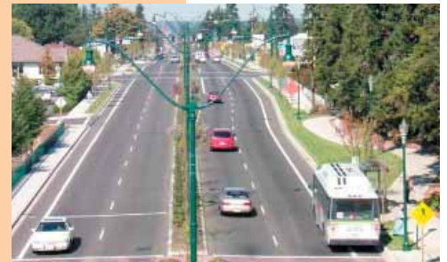
Bridgeport Way in University Place, WA before (above) and after (below) improvements were made.
