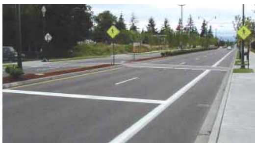
Advance stop lines can help prevent multiple threat pedestrian crashes.
