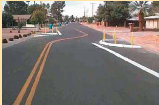
Traffic calming techniques, such as chicanes, were used in this targeted area to slow vehicle speeds on neighborhood streets.
